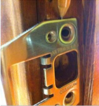
The lock should now fit flush on the inside of the door jamb. Do a test and close the door and see if the striker plate makes contact with the door. If it does not make contact, then you do not have to mortise the striker plate in the door jamb. If there is contact, even a little bit, then you must continue with step 20
