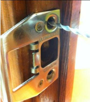
After the set screws have been installed, go ahead and proceed to pre drill the main screw holes with the drill bit that comes in the packaging. NOTE: Make sure you pre-drill the hole at least 3 ½ inches at a 30 degree angle in order to allow for the screw to go in without a problem. The screws are soft metal and will strip if not pre-drilled correctly.
