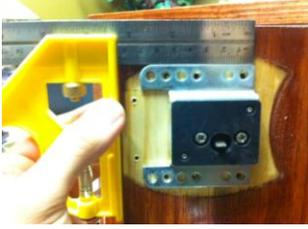
After the housing plate is snugly fit align it to make sure it is straight with your speed square. This makes sure the lock stays straight. Loosen the screws a bit to allow the housing plate to move more freely to allow for corrections in positioning. It is a good idea at this point to test and see if the gear goes in and out of the hole easily, if it does not loosen the screws and try again.
