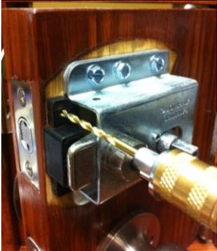
Place the shock absorber into opening of the lock (as seen on the left) and keep in place while drilling with a 1/8 drill bit. Make sure that the shock absorber is flush against the locking unit and pressed downward if there is a little wiggle room. **Note: When drilling be careful not to drill through the deadbolt lock, when you feel like you hit something stop drilling.**
