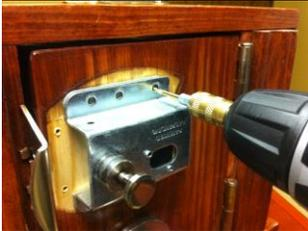
Place the platform plate on top of the housing plate and align them so the rounded corners match up perfectly. From here you pre-drill the 6 holes with the 1/8 drill bit. **Note: Be careful not to drill through the other side of the door.** Tip: You can also use a pencil or a hole punch to mark the holes and drill them without having to hold the platform plate in place.
