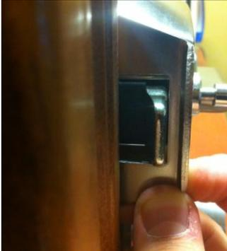
Place the striker plate on the door jamb and proceed to close the door. At this point try and align the striker plate where it is as close to the security bar as possible but not touching it. A good rule of thumb is that the striker plate and the security bar should not be more than 1/8 of space away from each other. Once you center and align the striker plate, mark its location with a pencil for placement location.
