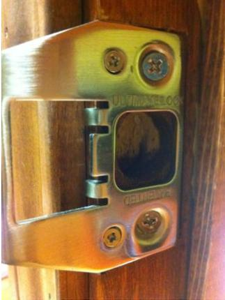
After you install the screws your striker plate should look like this. Go ahead and test the lock and make sure everything is running smoothly. Some things to check for can be: If the door clears the striker plate (no rubbing), the acceleration distance is perfect (see pictures), and if the lock opens and closes properly.
