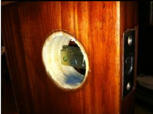
Install the deadbolt with the "up" arrow pointing up for left hand swinging doors and "down" for right handed swinging doors. Before adding the screws to hold it in place, make sure the deadbolt plate is flush with the edge of the door. If the bore hole is too big and the deadbolt plate sinks in then proceed to add 4 number 4 screws to create a surface for it to sit on.
