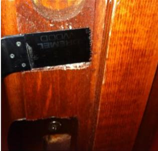
Mortis out the doorjamb with a cutting tool such as a Dremel multi-max, sonicrafter, or a wood chisel. Mortis out the hole for the strike plate enough were the striker plate and the door jamb are flush with each other
