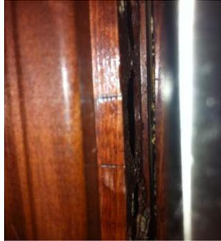
Open the lock, about 50%, just enough were the deadbolt hits the surface of the door jam. Once there mark the top and bottom of the deadbolt with a pencil. This creates to lines that will act as a guide for the striker plate you will install.
