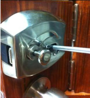
Install the small screws into the faceplate to hold it onto the rest of the lock. **Do not over tighten! This will cause the lock to open and close roughly! NOTE: Don't forget to record the serial numbers on the inside of the face plate and to input them on your control panel.**
