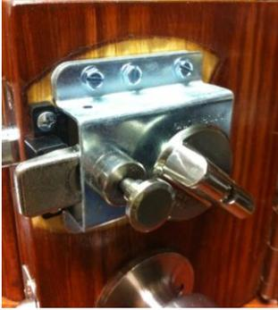
Test the lock by inserting the thumb knob on the lock and proceed to open and close the lock. If the lock is rough then try to pry the lock with a flat head screw driver a little bit. For instructions on how to do this please watch our install video.
