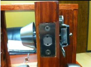
Insert the cylinder and housing with the 2 cylinder screws that hold it all together. **Note that the cylinder and the housing have to be installed upside down for right hand swinging doors.** Make sure that the two screws that hold it all together are **snug and not too tight**. Over tightening will result in a collapsed hole for the gear to go into making it almost impossible to unlock and lock at the completion of the install.
