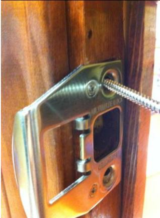
After you have pre-drilled the holes, proceed to install the main 3 ½ inch screws at a 30 degree angle. If you have a drill with a clutch installed on it set the clutch to about a 12 at low speed. Try to put as much force behind the screws as possible to avoid stripping. NOTE: The striker plate may be pulled back do to the install of the screws.
