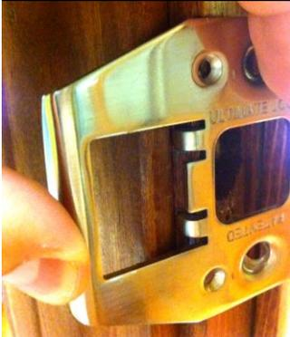
Place the striker plate on the surface of the door jam were the two lines that you drew line up perfectly inside the curved feet of the striker plate
