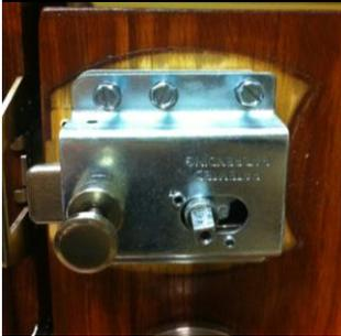
Set your power drill to about a 7 or an 8 torque and attach the 5/16 machine screw bit. From there go on to screw in all 6 #10 screws into the holes you pre-drilled earlier. **Note: For harder wood doors the torque may have to be upped a little bit.** Again proceed to check and make sure lock turns without any problems.
