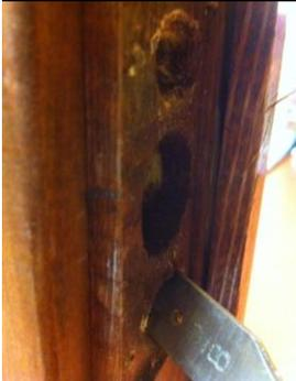
Using a 3/8 spade bit, or Dremmel tool, place it in on the marks you made on the inside of the main holes door jamb and dig into the wood enough that the dimples on the back of the striker plate sit flush on the door jamb.
