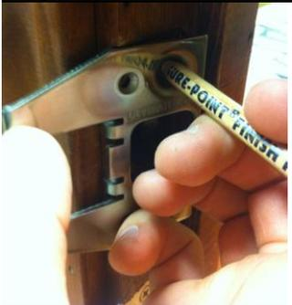
After placing and holding the striker plate firmly in place in between the two lines you have made. Grab a number 2 pencil and mark on the inside of the main holes.
