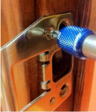
Go ahead and install the set screws into the lock in the position that you want it to stay in. It is important to note that before you install these screws that you pre-drill the holes either with a drill or with a hole punch.
